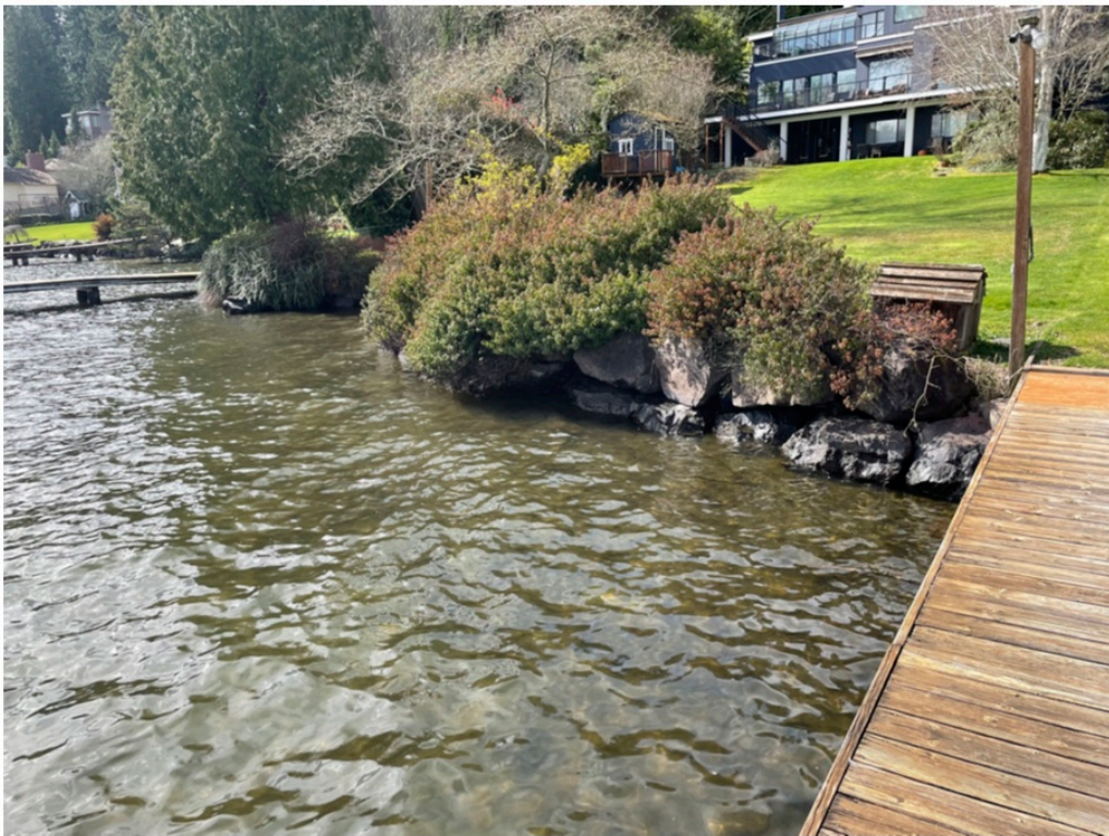
Photo 4 - Shoreline conditions looking landward on the south side of the existing dock.
