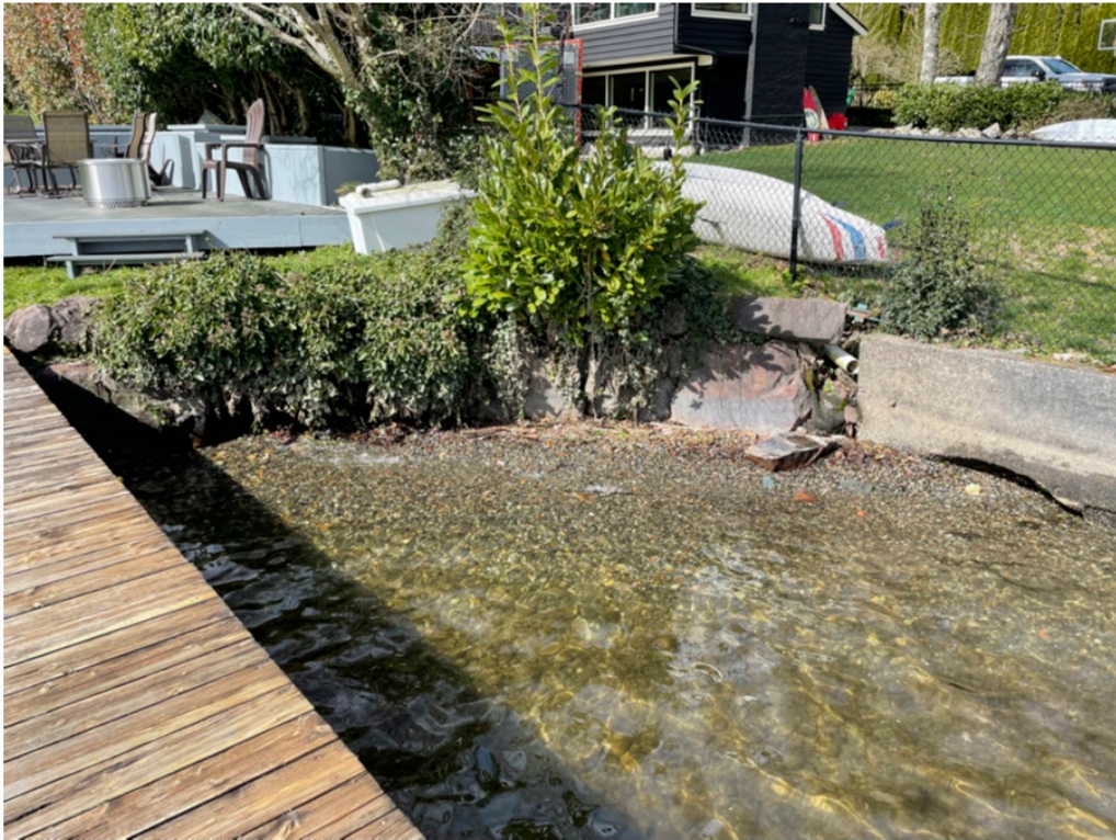
Photo 3 - Shoreline conditions looking landward on the north side of existing dock.
