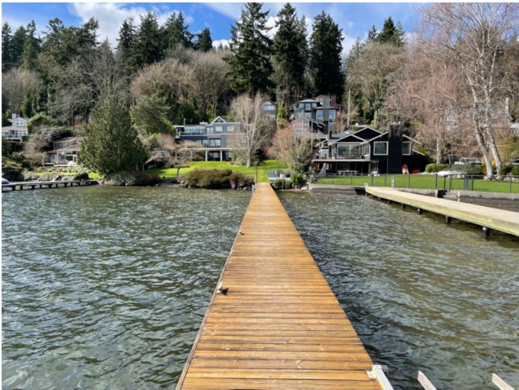
Photo 2 - Existing dock looking landward.
